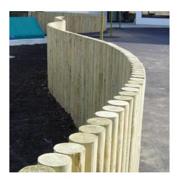
Log Walling forms a visually attractive yet effective barrier and is often used in parks and around play areas, where it blends well with other landscape features and planting. Log walls are formed from timbers between 75 and 150mm diameter, and are set in a concrete filled trench to ensure a strong and durable barrier is created. Log Walling can be used both as a barrier and retaining wall, and is suitable for a wide mix of leisure applications.
