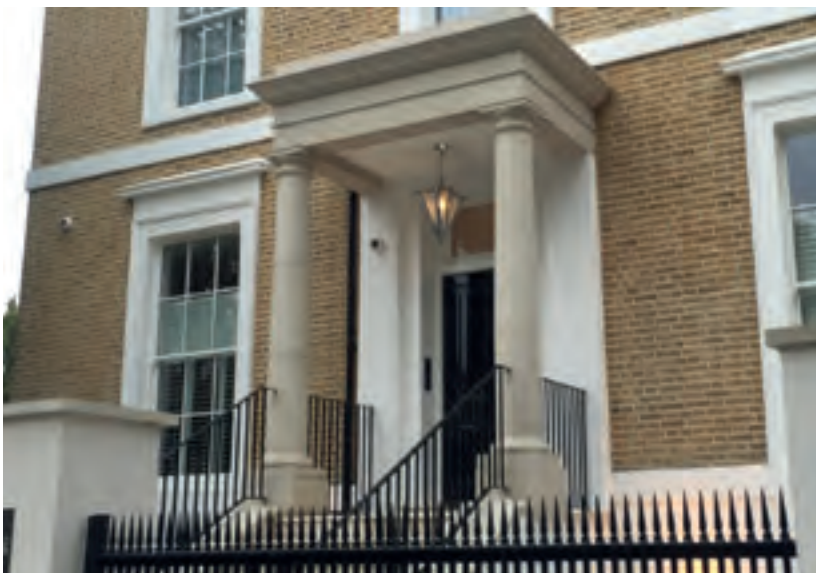
New portico on restored residential property
