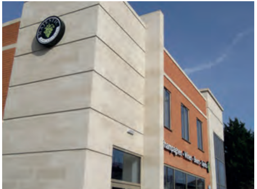
Ashlar walling on contemporary retail building
