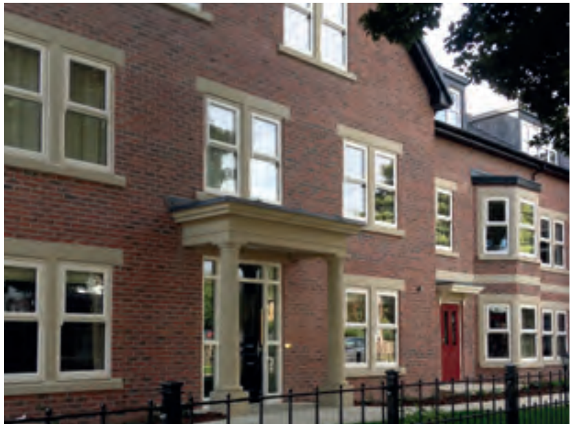
Portico, canopy, window mullions, cills and heads
