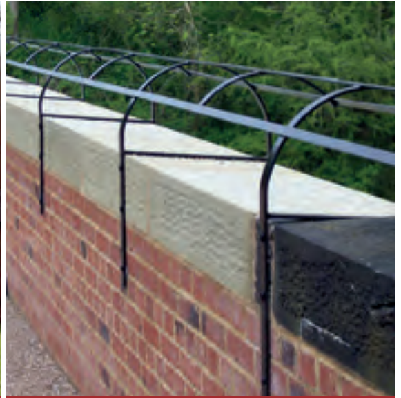
Wall copings on bridge restoration project
