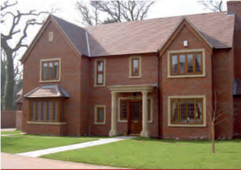
Portico, window surrounds and gable vent
