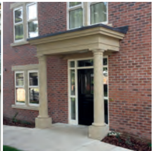
Portico on new residential property
