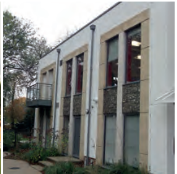
Window surrounds on contemporary residential building
