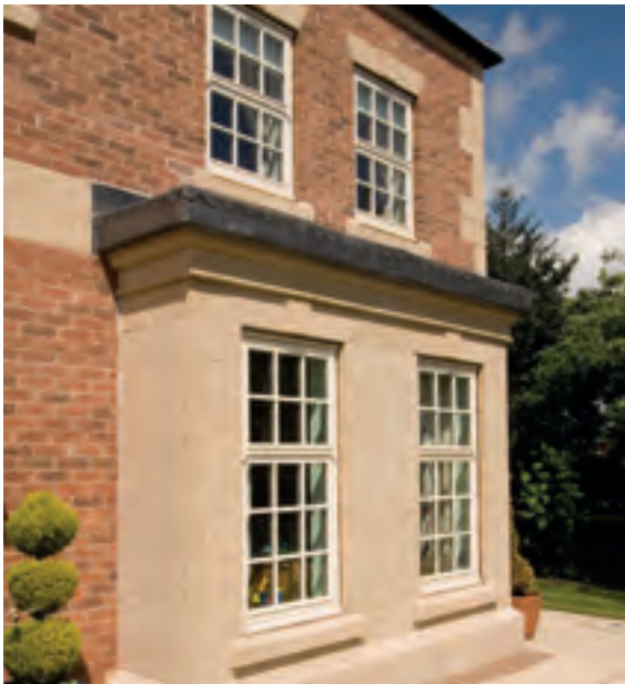
Ashlar walling, window cills & heads and quoins
